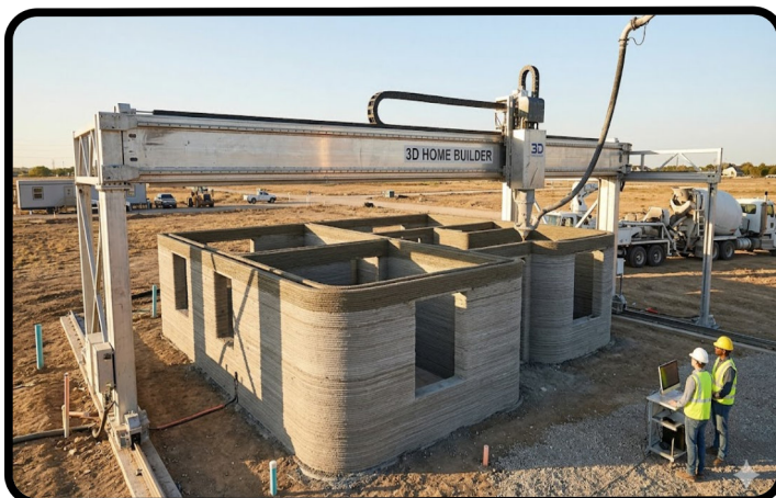
A house being 3D printed
